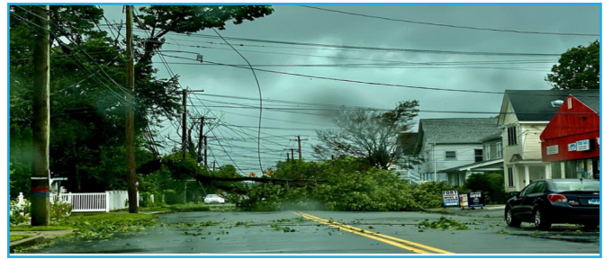
Damage to powerlines from tropical storm Isaias.
